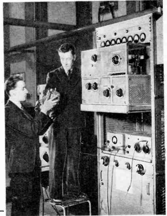
Experimental frequency modulation transmitter used at Alexandra Palace for the trials
